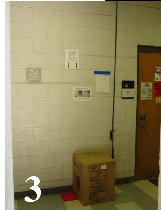
Loading Dock of NSC
